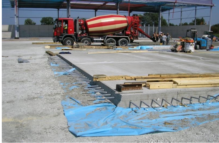
Establishment of the concrete floor
