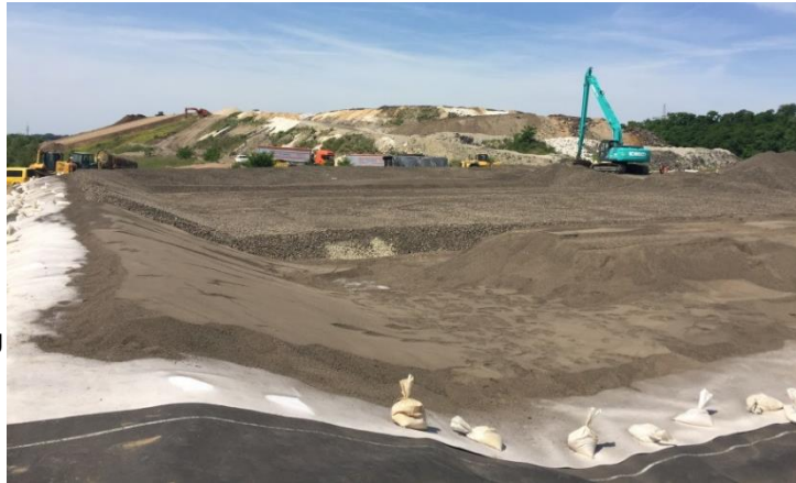
3 rd construction phase of the mineral landfill
