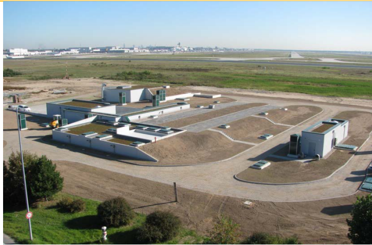
Rain water retention basin K
